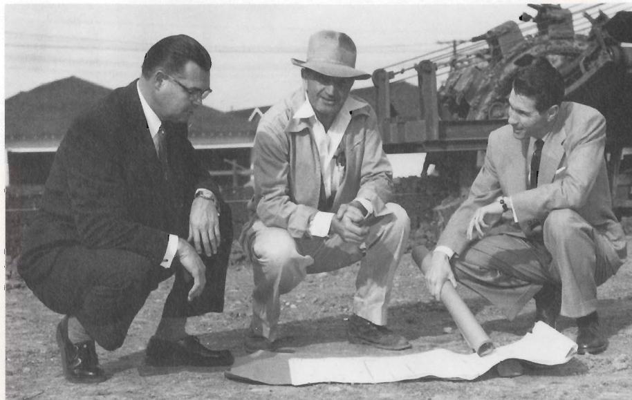
Bob (right) and Norm Neely (left) meet with a contractor in 1953 to finalize plans for the Neely headquarters at 3939 Lankershim Boulevard in North Hollywood, California.
